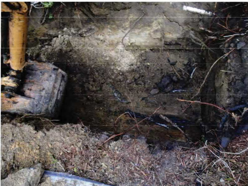
Picture 2: UST 781LaurelBB excavation in progress.
